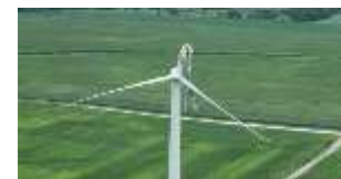
Wind Blade Damage by Fierce Strom
