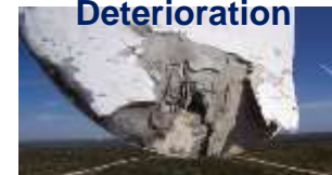
Blade Tip Damaged by Lightning Strike
